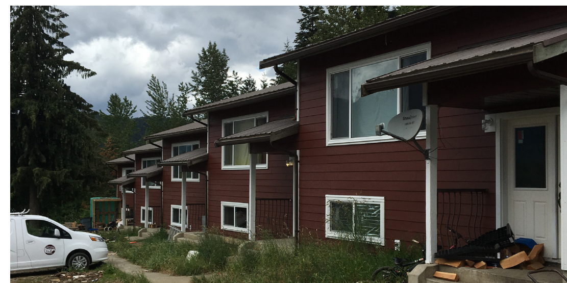
ISTKEN LANE, 2 BDRM ROWHOUSES, BUILDING ENVELOP RENOVATION
